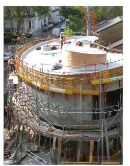
The external staircase has been designed as a curved RC structure supported on RC columns due to the shape.
